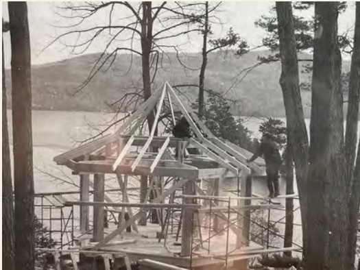
Tea House under construction 1972.
